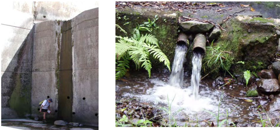
Figure 8. Vertical drop as a barrier on ‘Īao Stream, Maui (left) and a pipe providing for water flow downstream over a diversion on Hanehoi Stream, Maui. While not actual stream diversions, the images show potential obstacles that animals migrating upstream may encounter. Notice the extent of the drop in comparison to the normal channel gradient in left image. In the right set of images, it is unknown if hydraulic conditions (too swift or turbulent flow) or the unsuitable substrate (smooth pipe may prevent animals from holding on to pipe sides) would prevent upstream migration. Additional behavioral issues may also be a factor in the extent of fish passage through the pipe (fish may avoid dark areas).
