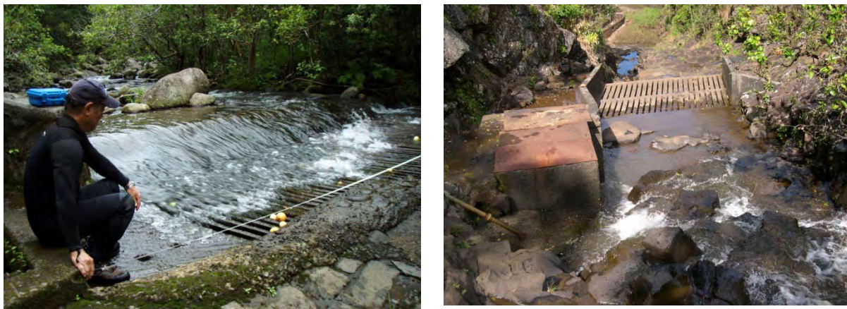
Figure 19. Stream diversion intakes on Waihe'e Stream (left) and Honopou Stream, Maui (right). Notice how 100% of the water flows into the diversion at this discharge. An animal moving downstream would be transported with the water and entrained in the diversion structure resulting in 100% mortality.
